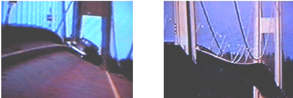
Figure 1.1: (left) View of Tacoma Narrows Bridge along deck; (right) view of torsional vibration
