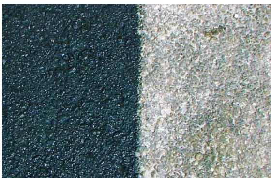
After Seal Coating
