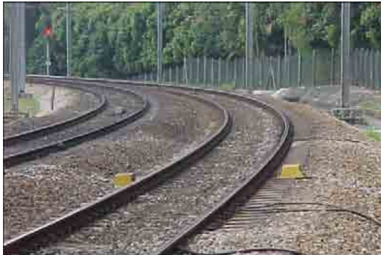
Track magnets mounted outside the rails at the approach to a neutral section in 25 kV AC catenary. Detectors carried on the leading bogie switch off the power supply on the train as they pass over the magnets. On the other side of the neutral section, a second set of magnets switches the power on again.
