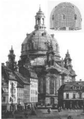
elastic-plastic Masonry Analysis of the Church of our Lady in Dresden
