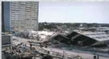
1985 MEXICO EARTHQUAKE: NUEVA LEON APARTMENT BUILDINGS
