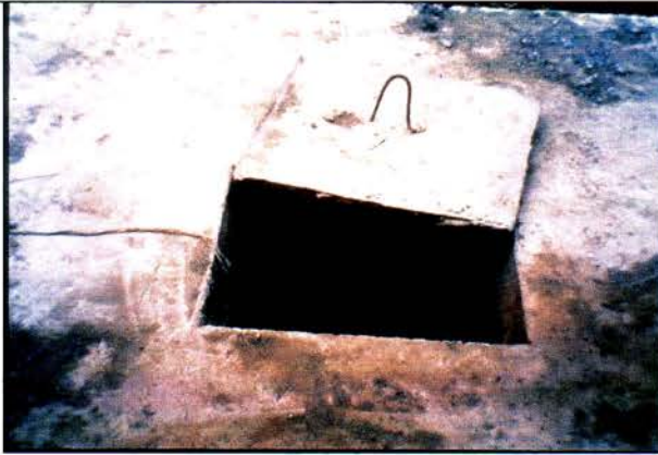
Two Compartment Septic Tank
