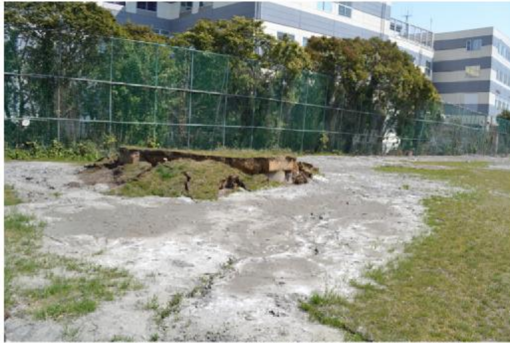
Figure 7. Uplifted tank in a park field in Urayasu (N35.6398, E139.8235).
