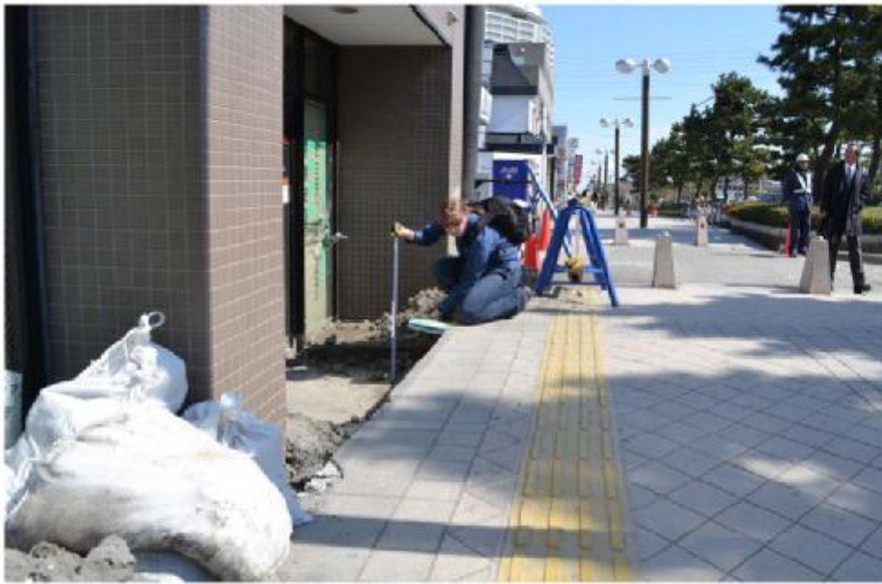
Figure 5: Sidewalk settles relative to a building on piles (top left), whereas a three-story building settles more than the adjacent sidewalk surface (top right, and bottom) in Urayasu (N35.6485, E139.9178).
