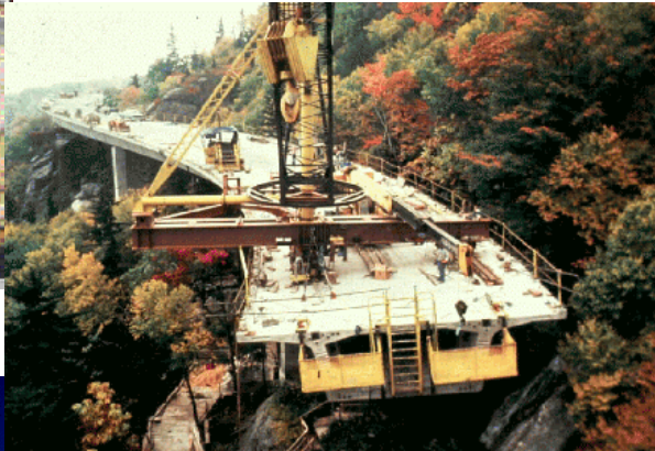
Note the use of trapezoidal box girders
