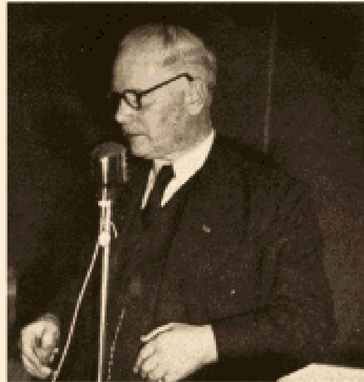
Professor Magnel teaching prestressed concrete.
