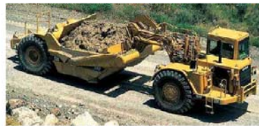
Hauling excavated soil
