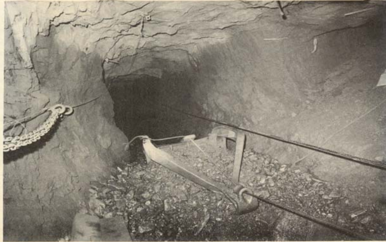
Scraper loader bucket in a scram drive. Mill hole in foreground, drawpoint on right. (Courtesy Joy Manufacturing Co. Pty Ltd)
