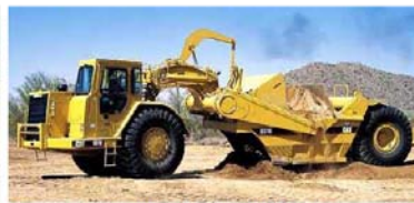
Discharging bowl, spreading soil
