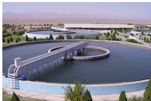
Flocculator-clarifier provides mixing, flocculation, & sedimentation in a compartmented concentric circular tank.
