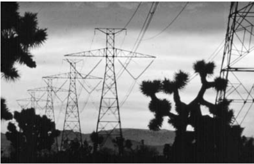
Figure 2 A \pm 500 -kV HVDC transmission line
