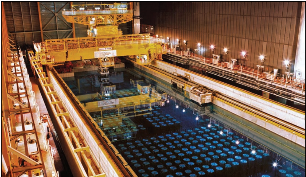
At a nuclear plant in England, barrels containing radioactive waste are stored in a pool where they are kept cool.
