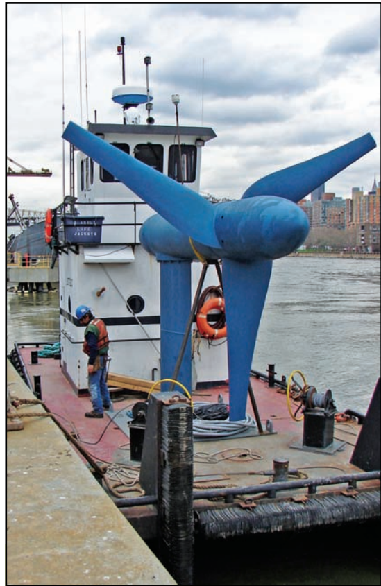
Workers prepare to install an underwater turbine in New York City's East River in December 2006.
