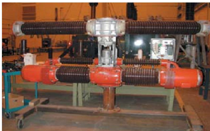
DLF air-blast breaker module
